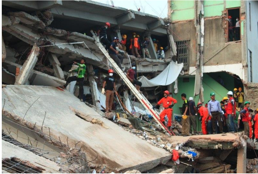
Figure 2: Rana Plaza's collapsed building
